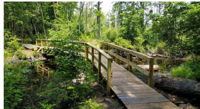
Wooded Boardwalk and Bridge
